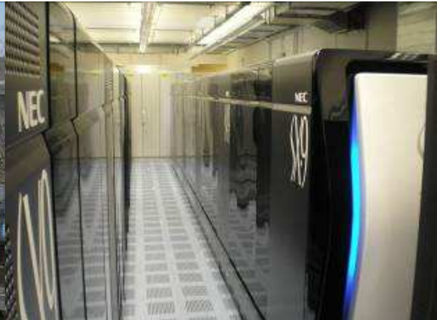
Machine hall with NEC SX-9 Supercomputer
